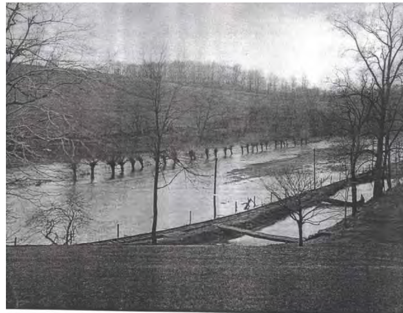
Figure 5. This picture appears to be taken about the same time as the one in figure 4 (possibly the same winter). Here the flood plain meadow has been flooded by the Red Clay Creek but the trolley tracks are above the water indicating the trolley roadbed was on a grade level somewhat higher than the meadow. Photo Credit - Hagley Library and Museum
