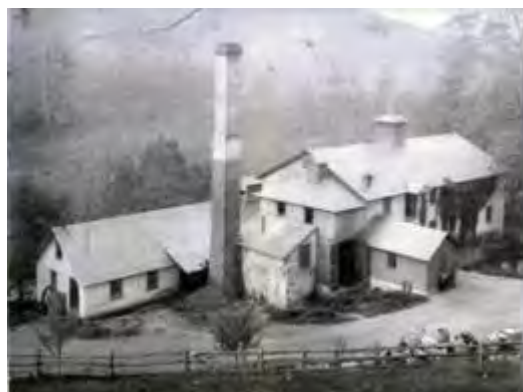
Thomas S. Marshall & Sons Paper Mill, Marshall's Bridge, Pennsylvania, 1880s. The section to the left along with the stack and the small addition toward the road were torn down when the mill ceased operation about 1910. The remaining portion now features two townhouses, complete with waterwheel.
